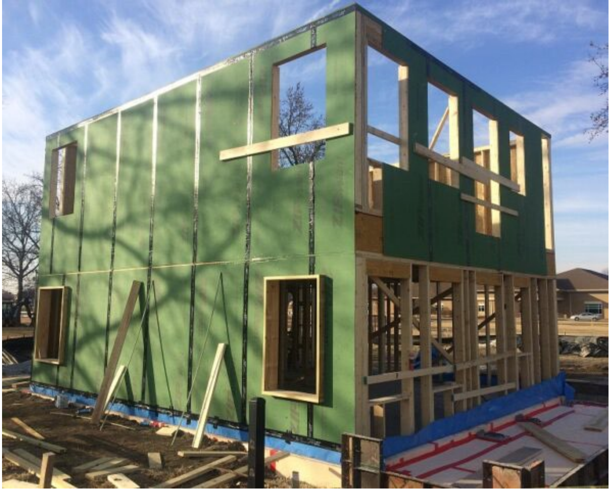
GCHA - Construction Photo by Tony Holub
